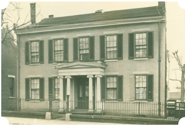
Original Wheeling Hospital Location on 15th street.
