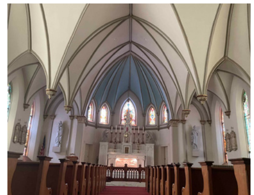
Inside St. Peter's Church in Harpers Ferry, WV, where work is being done to prevent the sacred walls of the church to slip away from its foundation.
